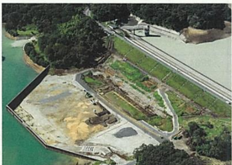
① Before reinforcing dam body (September 2020)
