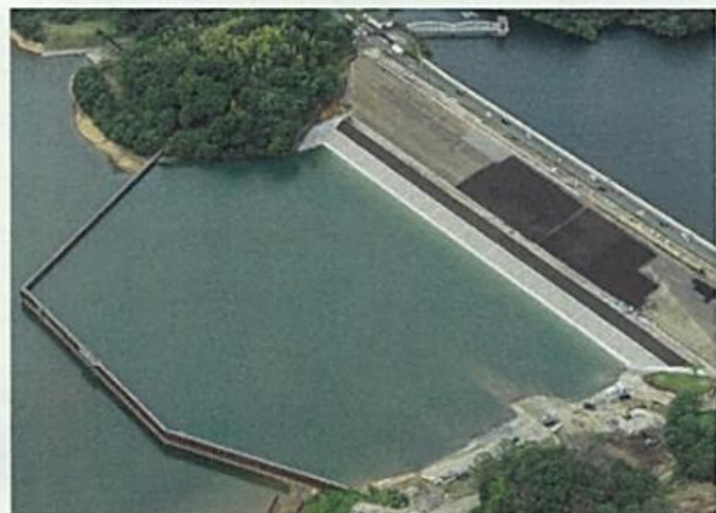
⑤ Implementation of initial impoundment (high water level) (June 2023)
