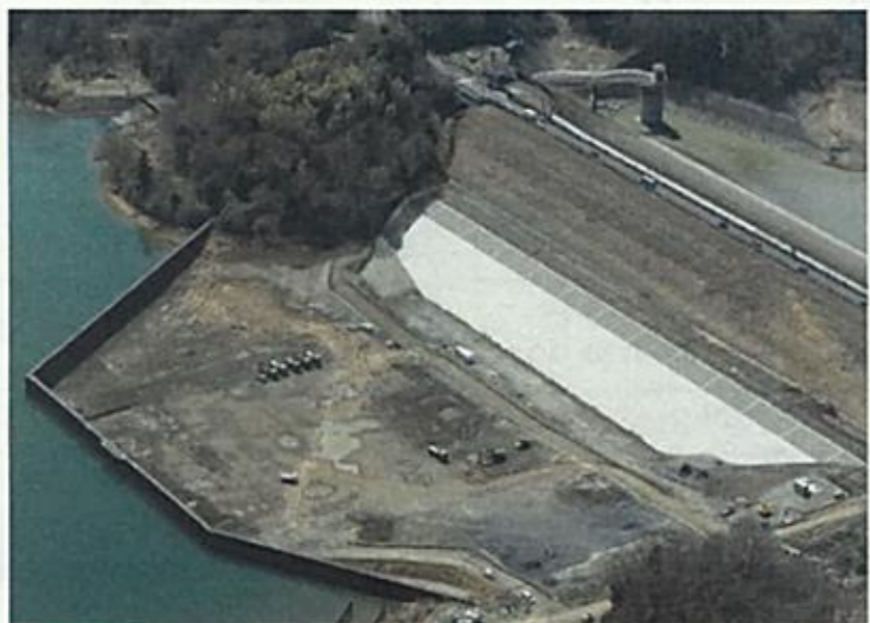
④ Complete view upon completion of building-up (February 2023)
