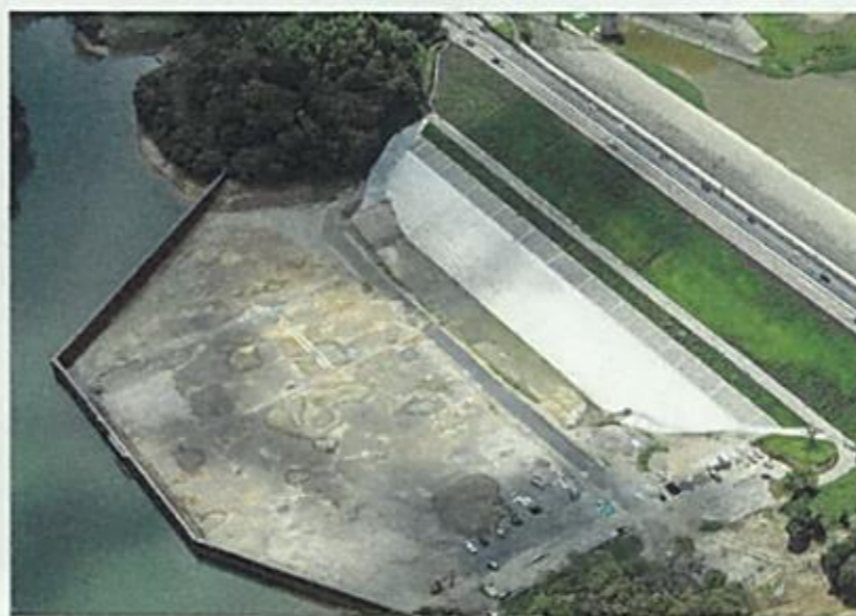
⑥ End of initial impoundment; completion (August 2023)
