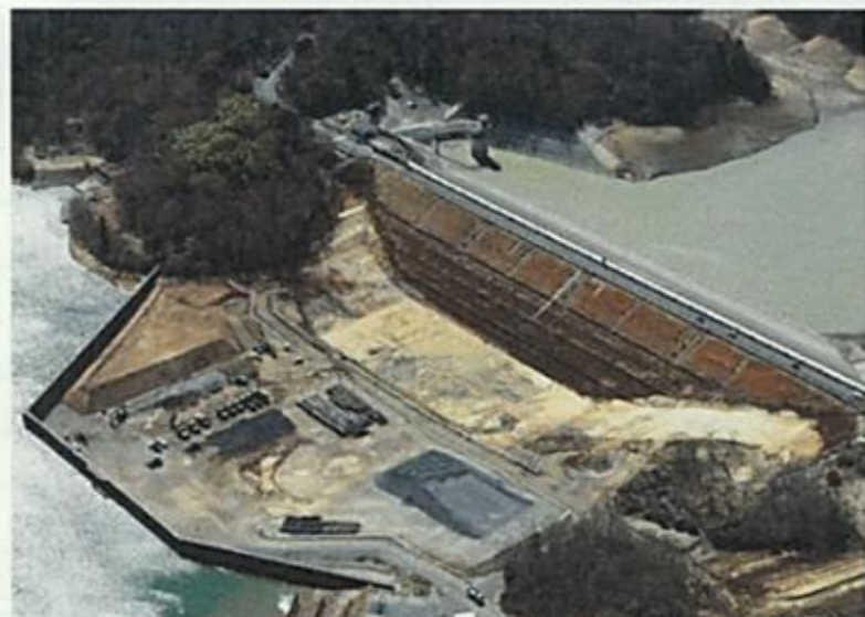
② Excavation of existing counter weight berm fill (March 2021)
