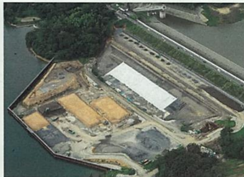
③ Building-up of reinforcing embankment fill(September 2022)
