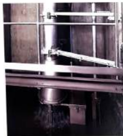
Wastewater pre-screening in the intake structure with a HUBER Pumping Stations Screen ROTAMAT® RoK4.
